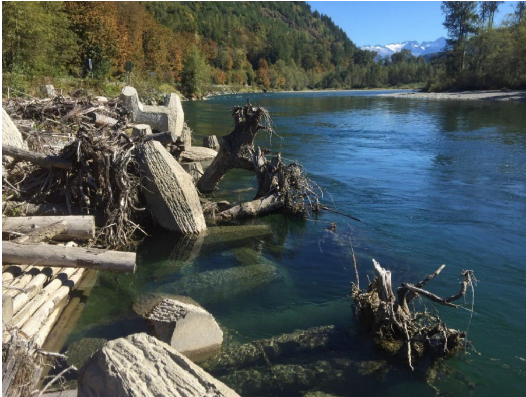
Figure 10A-9 Dolotimber Structures, Skagit River, Skagit County
