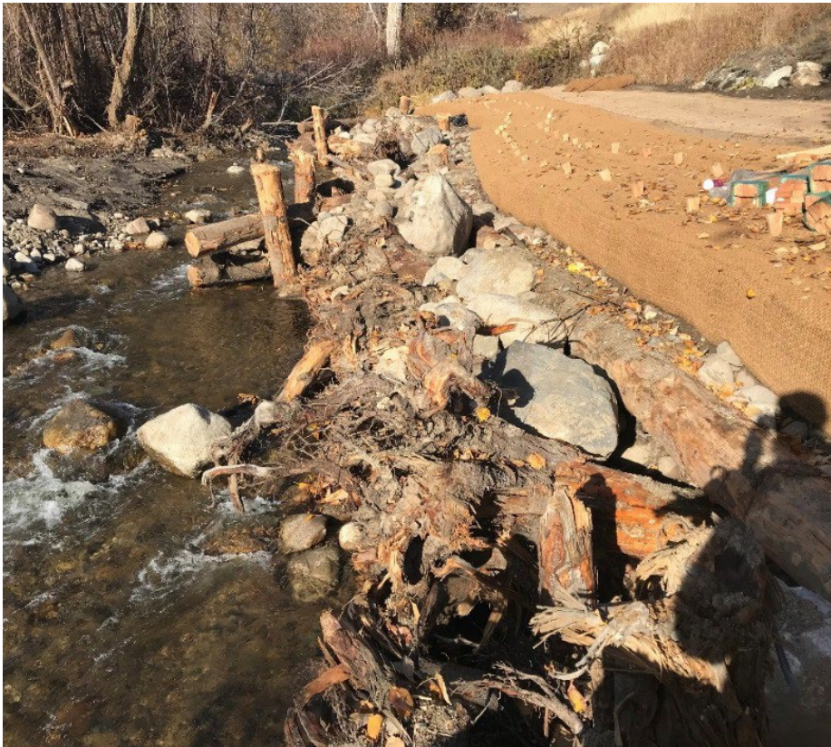
Figure 10A-4 Crib Wall with Wood Piles, Beaver Creek, Okanogan County
