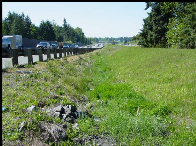
Continuous Inflow Biofiltration Swale along I-5 in Snohomish County
