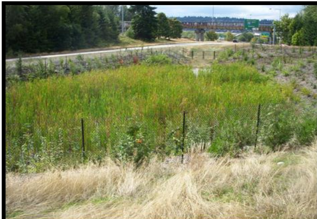
I-405 Bellvue Combined Stormwater Treatment Wetland/Detention Pond
