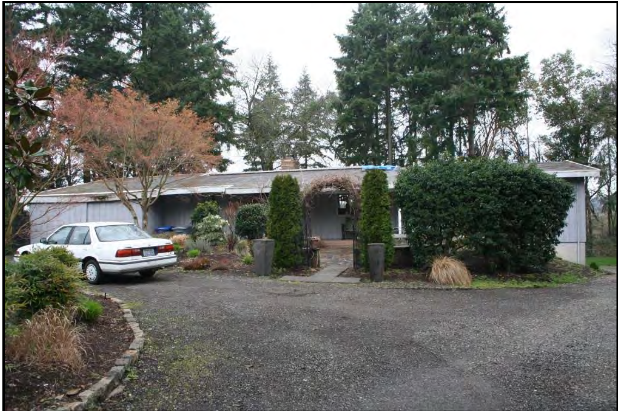
Figure F.6. Cerna House, 11610 SE 45 th Place, east elevation, view to the west.
