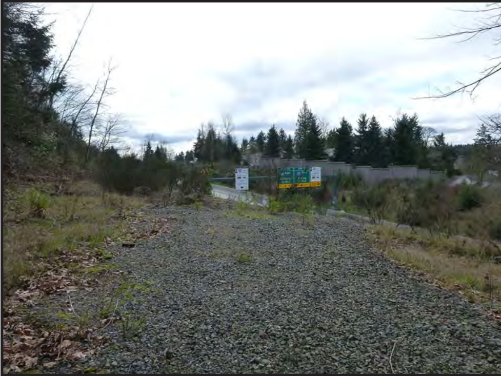
Figure 62. Overview of the former Wilburton Tunnel location in 2016, view to the southwest.
