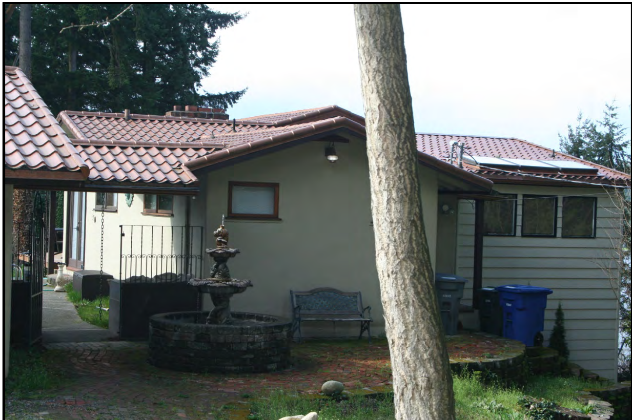
Figure F.8. Garcia House, 5449 Lake Washington Blvd. SE, east elevation, view to the west.
