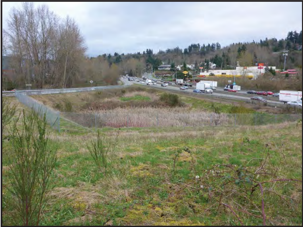
Figure 19. The storm water retention pond located in Zone 38 is shown in this photograph to the northeast.
