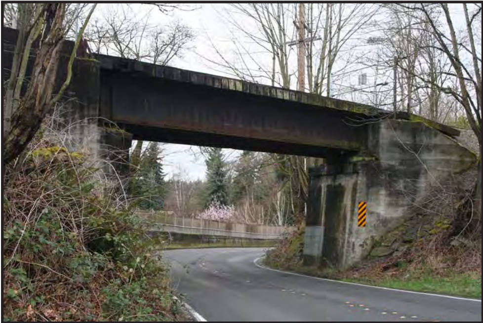
Figure 46. Lake Washington Boulevard overpass, view to the north.
