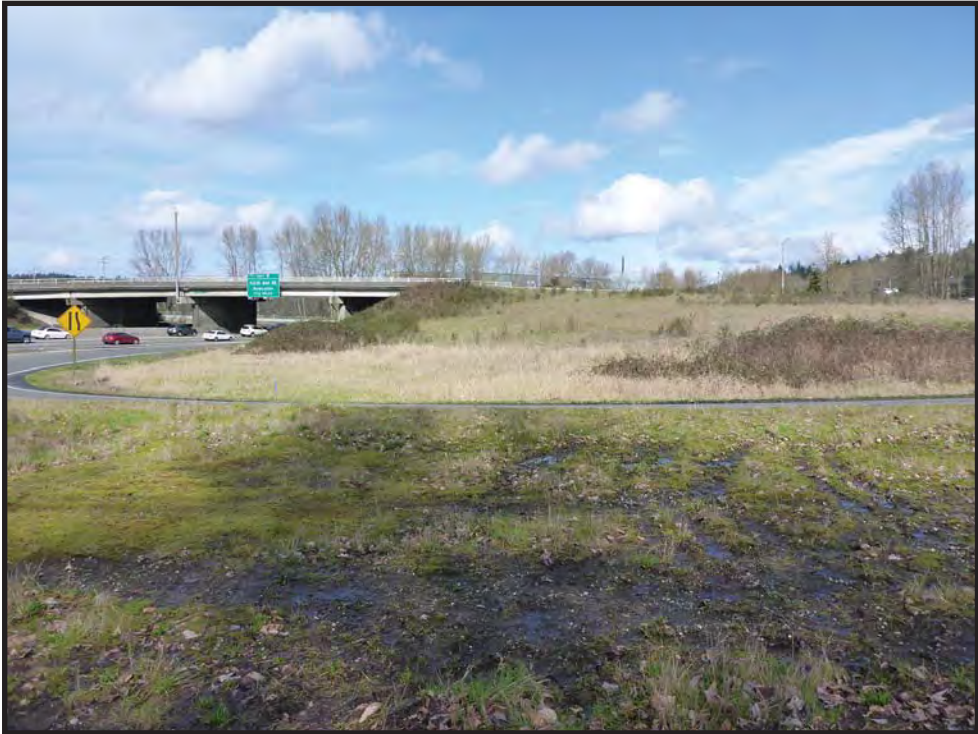
Figure 12. Zones 33 and 34, two traffic islands in the southeast corner of the NE 44th Street interchange are shown in this photograph to the north. Zone 33 is in the foreground and Zone 34 is in the background.
