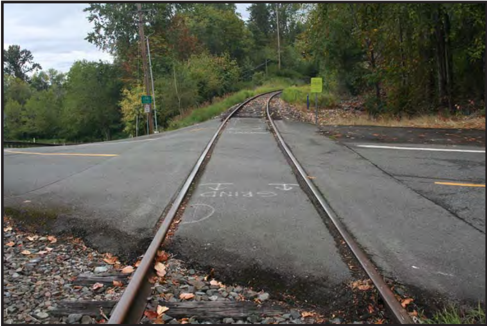
Figure 52. Grade crossing at Lake Washington Boulevard, view to the northeast.
