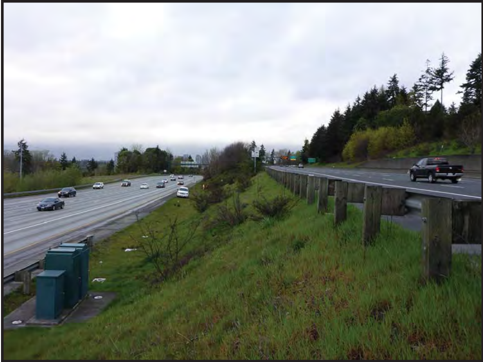
Figure 35. Overview of Zone 69, the paved lanes of I-405 extending north from the I-90 interchange at MP 11.30 to the north end of the project resource evaluation area. The crew is excavating ST 156 in this view to the north.
