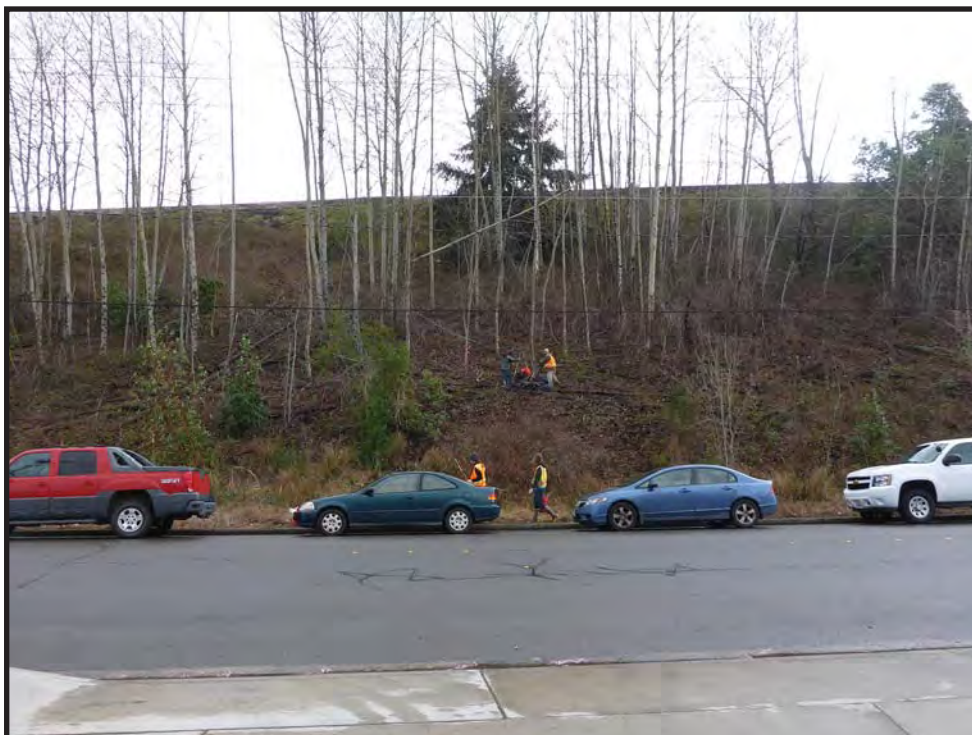
Figure 3. Crew excavating ST 16 in Zone 5. Shovel tests were excavated on the fill covered slope between the Houser Way bypass and I-405 southbound lanes. View to the east.
