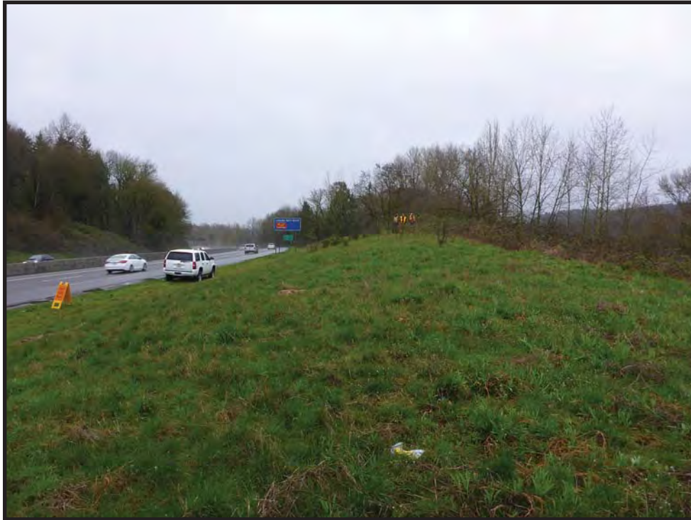
Figure 14. A large fill berm west of I-405 near MP 8.85 in Zone 35 is shown in this photograph to the southwest.
