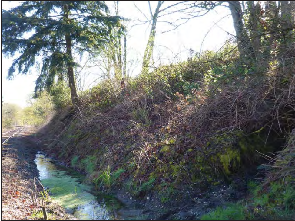
Figure 26. Portion of Zone 49 bordered on the west by the railroad grade. The crew is excavating ST 184 in this view to the northeast.
