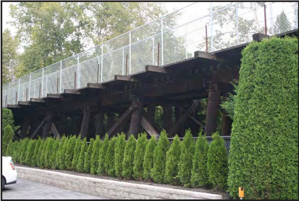
Figure 59. Ripley Lane trestle, view to the southwest.
