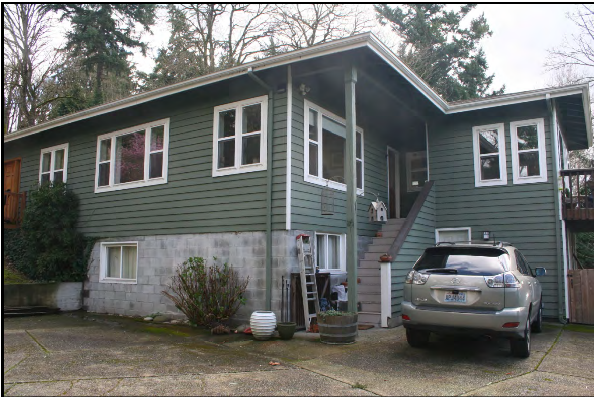
Figure F.7. Andrade House, 6633 Lake Washington Blvd. SE, north and west elevations, view to the southeast.
