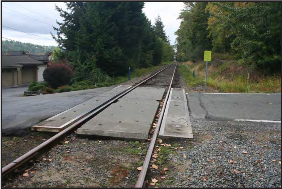
Figure 57. Grade crossing at Hazelwood Lane, view to the north.
