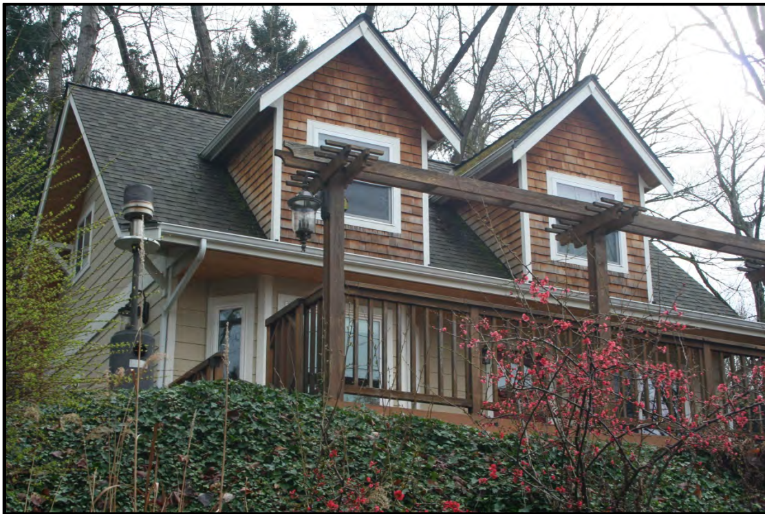
Figure F.2. Morriseau House, 4256 Lake Washington Blvd., west elevation, view to the southeast.
