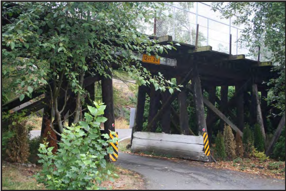
Figure 58. Ripley Lane trestle, underpass, view to the north.
