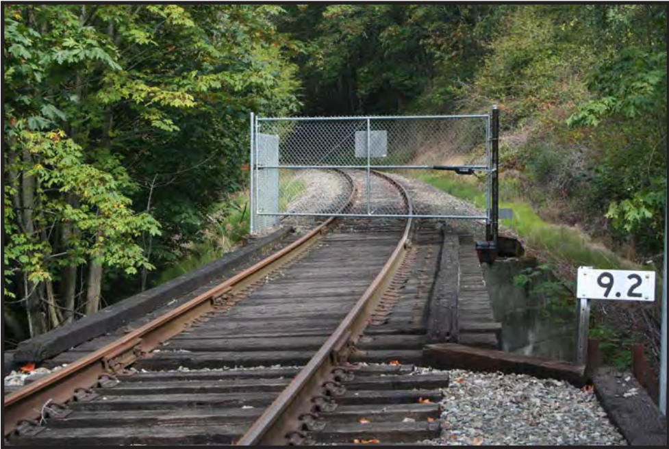
Figure 47. Lake Washington Boulevard overpass deck, view to the northwest.
