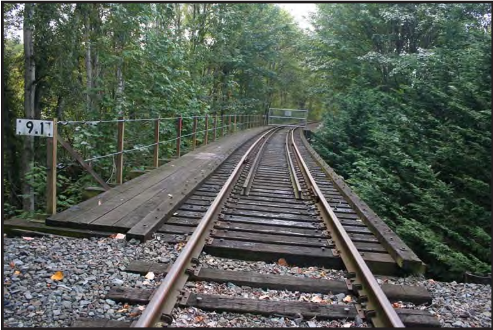
Figure 51. Coal Creek trestle, deck, view to the northeast.
