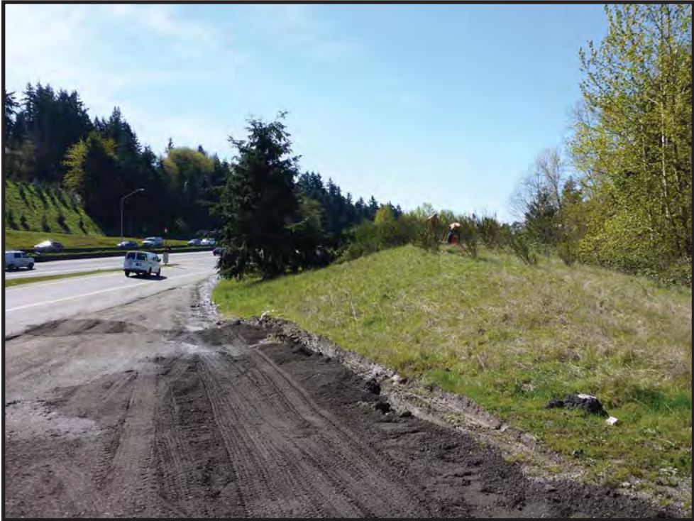
Figure 25. Zone 48, a linear earthen berm, is similar to the berm at the north end of Zone 35 (see Figure 14). View to the southwest.
