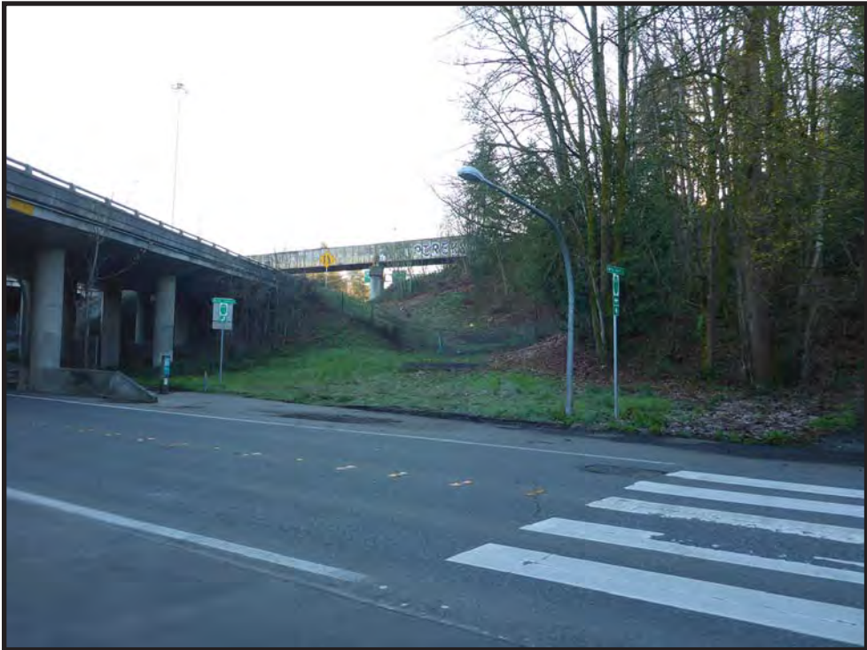
Figure 34. View from Lake Washington Boulevard showing an I-90 overpass to the left and the Northern Pacific Lake Washington Belt Line steel bridge crossing I-90 in Zone 65, view to the east. The utility vault is visible in the grassy area south of I-90.
