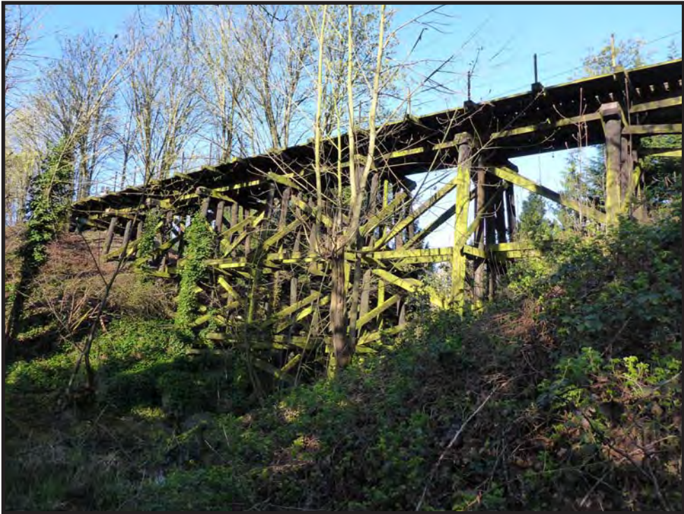
Figure 50. Coal Creek trestle, view to the northwest.
