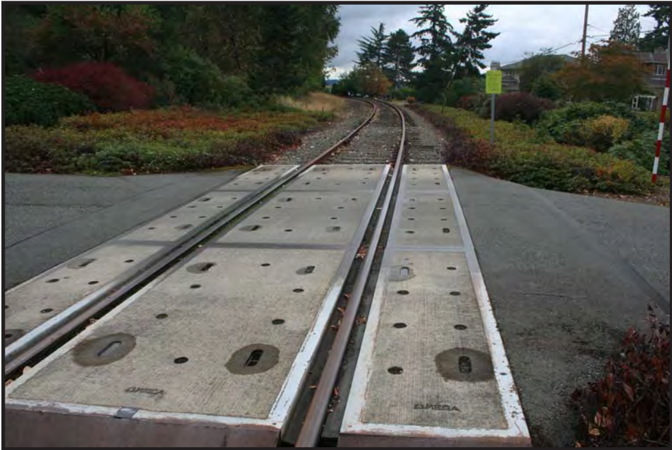
Figure 56. Grade crossing at Pleasure Point Way, view to the northeast.
