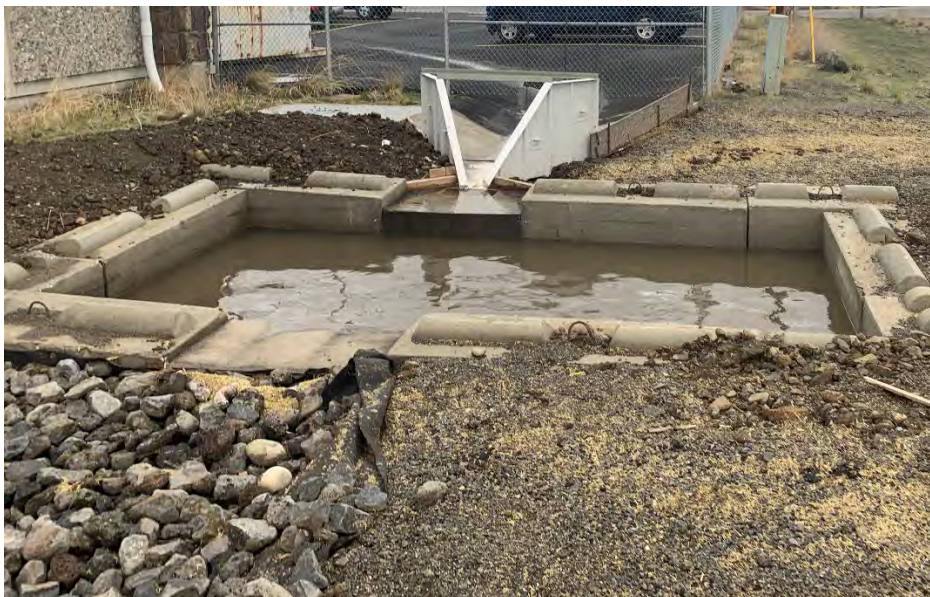
Figure 10 Geiger Influent with Siltation Basin
