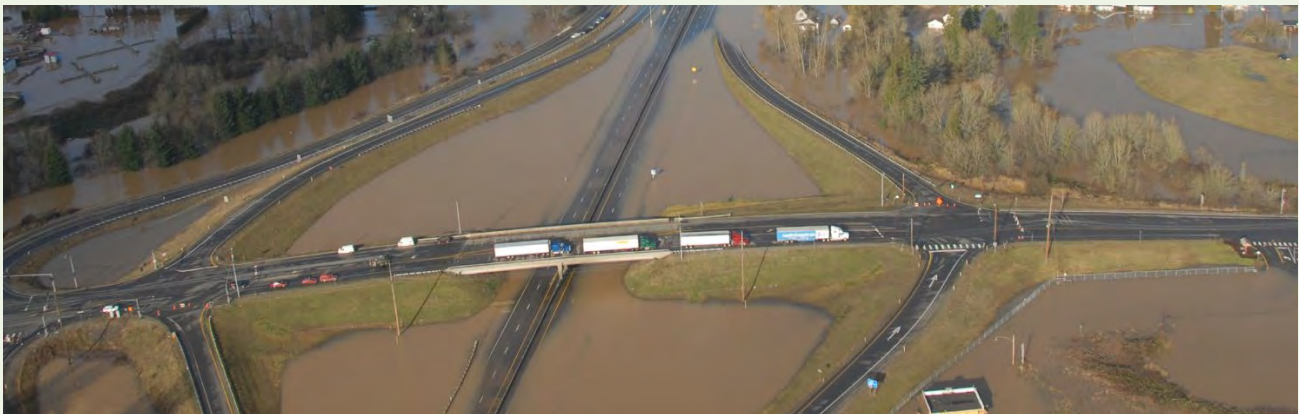
Figure 33: I-5 Flooding in Chehalis
